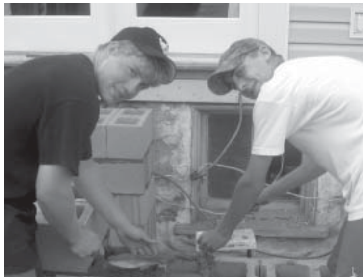
Two young PACE volunteers repair a flood victim's brick wall.
